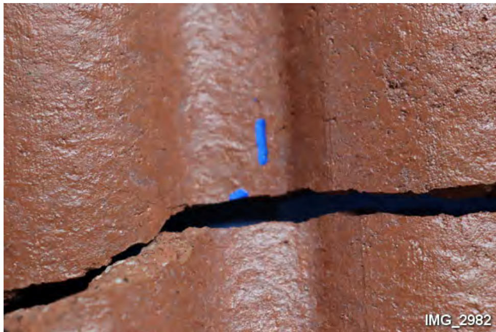
G19. Close-up of Impact 1. (Note impact broke tile.)
